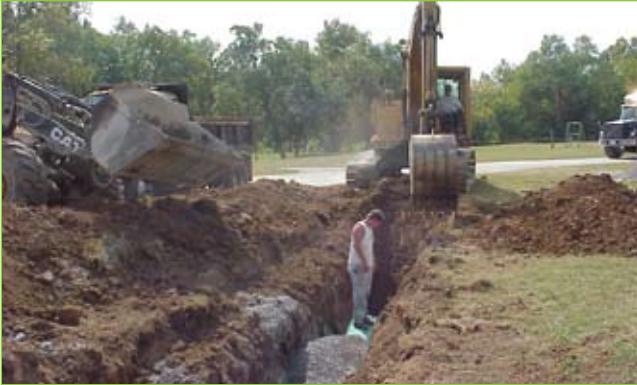
Development in the I-435 Corridor is dependant upon major infrastructure and utility investments. Pre-planning and coordination across jurisdictions is necessary to ensure utilities meet current needs and accommodate future growth.
